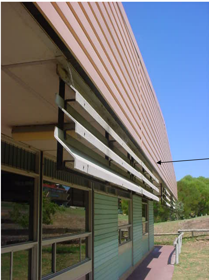
Asbestos cement sunshade louvres, fascia and wall panels
