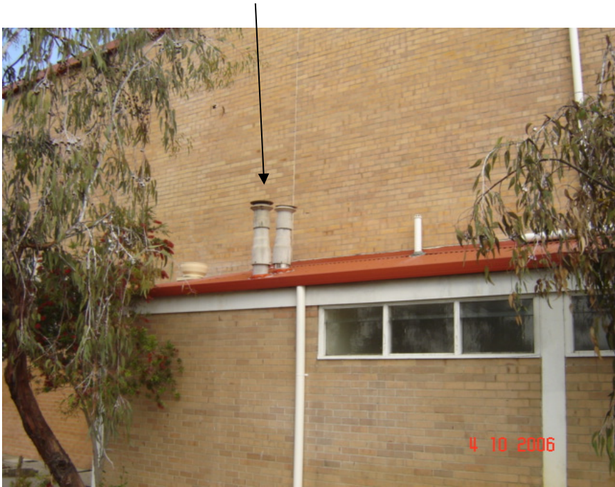
Asbestos cement flues
