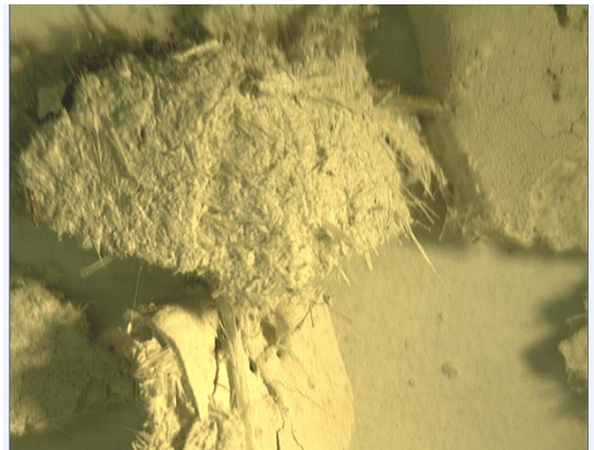
Low density board with brown and white asbestos.
